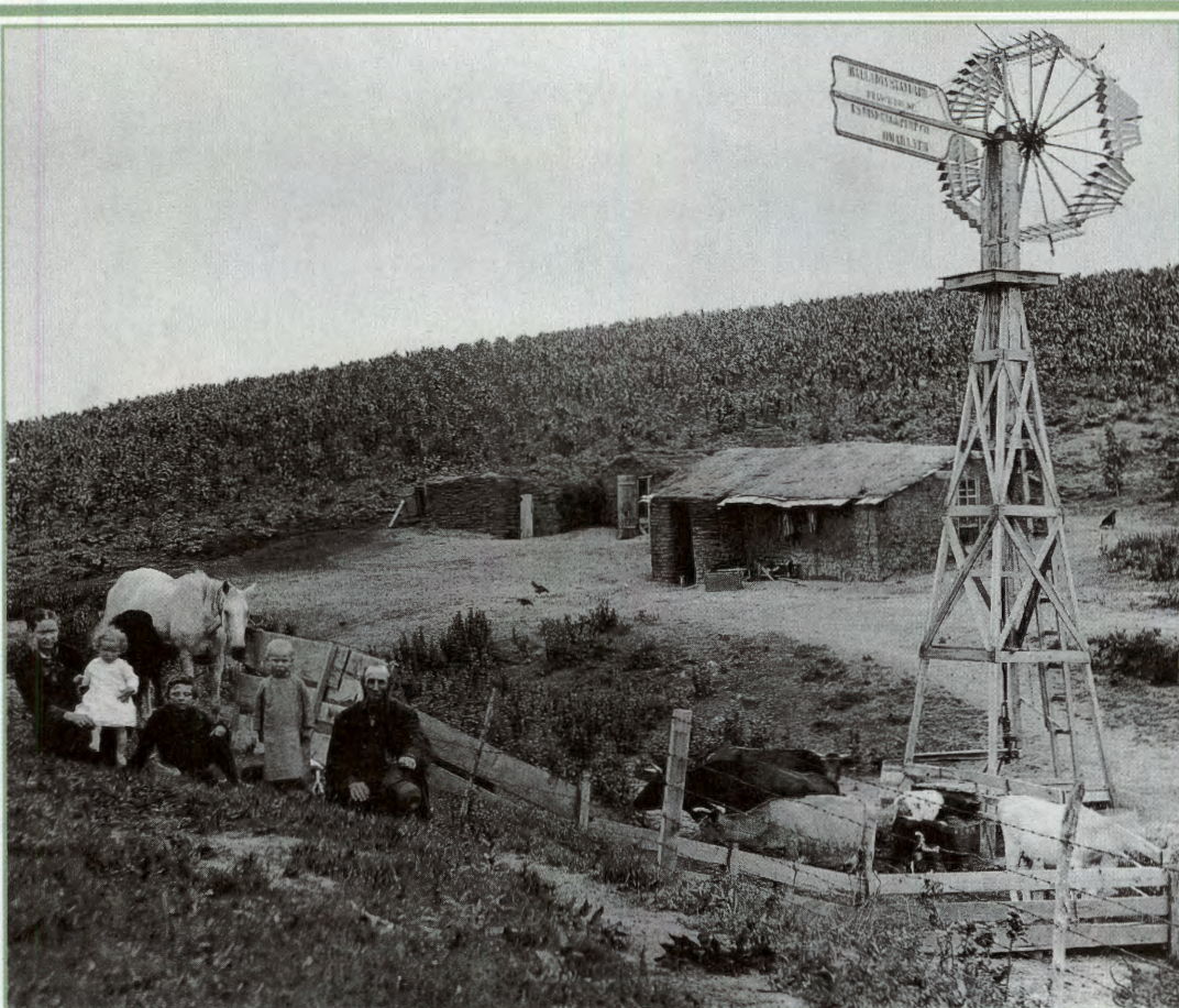
Windmills built over wells pumped water to the surface and also showed travelers where houses were located.
